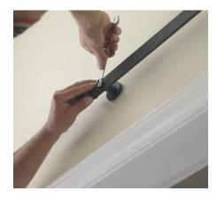
Using the flanges and screws provided by the manufacturer, **attach the rail to the wall.** The rail installation process may vary by manufacturer, so be sure to follow the instructions provided.
