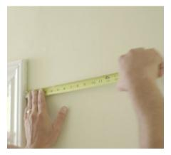
First, **ensure you have enough wall space** adjacent to the doorway where the door will slide. Be sure to determine the position of the doorstops, as they need to be slid on the rail before mounting it on the wall. The door stop will help ensure the door does not come off the rails while sliding.
