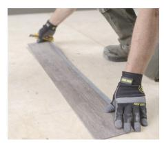
To cut a plank simply **measure and mark the plank,** then using your straight edge and utility knife, score the plank and snap.
