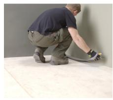
Starting from a corner, **install the first row with the under-edge facing away from the wall,** allowing a gap of at least 1/4" for expansion, which should be covered by moulding. Trim off the long side top over-edge facing the wall. Be sure to get the entire length of the first row as well as the overedge on the short side of the first plank.
