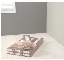
Begin by **laying out your unopened boxes of planks** in the room where they will be installed at least two days before you start, so they can acclimate to the temperature and humidity.
