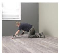
After installation is completed, we recommend **rolling the seams with a floor roller** in both directions to insure bonding of both adhesive edges.
