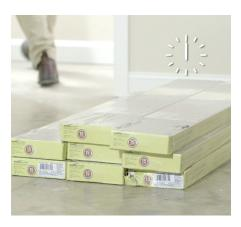
Lay out the unopened boxes of planks in the room where you will be installing for at least two days before you start, so they can acclimate to the temperature and humidity.
