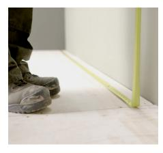
Figure out how the entire floor will lay out in order to **ensure the planks on either side of the room are similar in size.**
