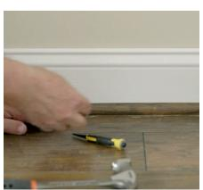
Once all the laminate flooring has been installed, finish up by **installing** matching thresholds and quarter-round moulding to the walls using finishing nails.
