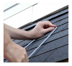
**Roof heating cables** will help you avoid long-term damage caused by freezing and ice build-up. Before installing the cables make sure your eavestroughs and roof have been cleaned thoroughly. Affix roof cable clips to your roof in a zigzag pattern. Finally, attach and secure your heating cable to the clips.
