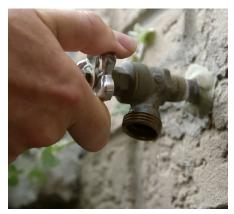
**Turn off all exterior faucets** and drain water from outdoor pipes, valves and sprinkler heads to prevent pipe bursts. If your home is 10-years or older, consider installing frost-proof faucets, available at The Home Depot.
