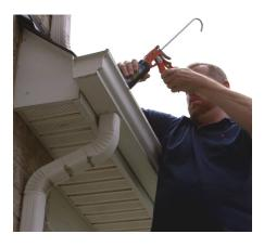
**Prep your eavestroughs and downspouts** by sealing any cracks with a silicone sealant and installing a filter to prevent leaves from clogging.
