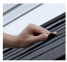
**Apply roof repair glue** to any loose shingles in order to help avoid leaks or damage. The Home Depot has a full selection of roof adhesives to choose from.
